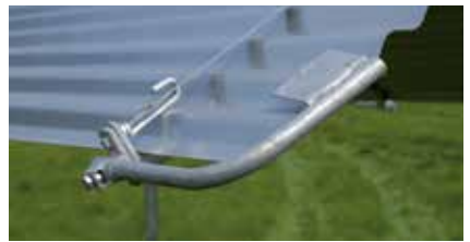
Corner protection for the roof
